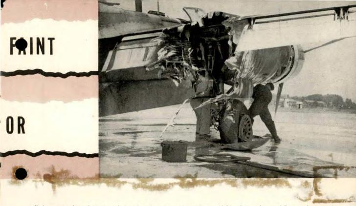
roll there was a loss of power and the odor of gasoline became stronger. The pilot decided not to complete his takeoff and slowed down to a stop at the end of the runway, then pulled over to a taxi strip to clear the runway for other planes. Upon doing this, his engine loaded up and stopped firing. Mixture control was moved from RICH to IDLE CUT-OFF and the engine started running again. The pilot advanced the mixture to AUTO-LEAN.
